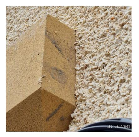
Location: Stoneworks Excessive mortar and render staining
