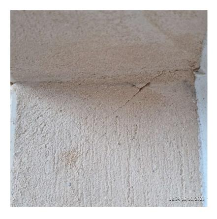
Superstructure Location: Bed 1 Cracking to rendered reveals
