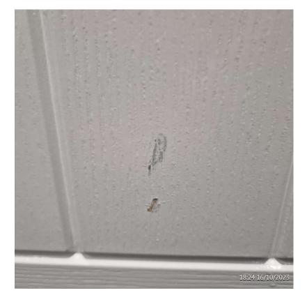
Location: Master Bathroom Damage to bulkhead sill lip
