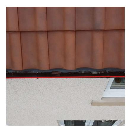
Unsatisfactory Location: Rear Guttering Debris found in rear gutter line
