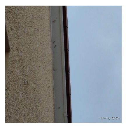
Location: Fascias And Soffits Excessive mortar and render staining
