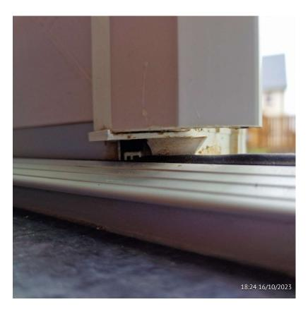
Location: French Doors Damage to bottom of centre mullion cap
