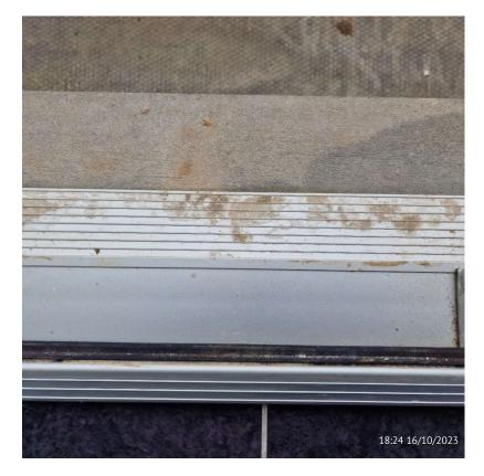
Location: Front Door Damage to leading edge of slab
