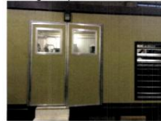
Mounting doors & intake louvers
