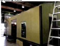
Closing building walls and framing
