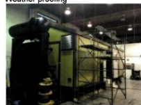
Finishing flashing work
