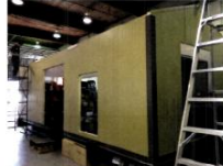
Closing building walls and framing
