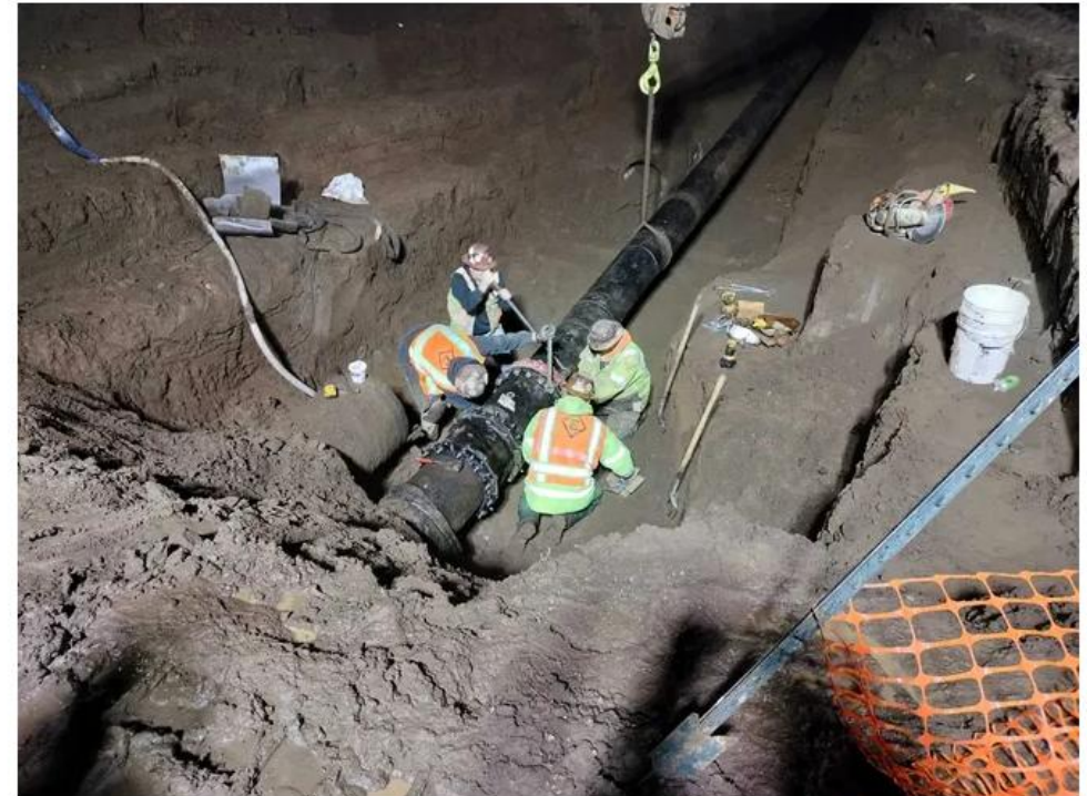
Salem Public Works crews worked overnight in late December to repair a 400-foot section of corroded pipe that disrupted wastewater service to West Salem. Provided By The City Of Salem
