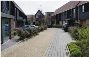
Contrasting permeable block paving used to reduce the apparent carriageway width, and reduce traffic speed, without impeding access by emergency vehicles. (Slow Streets Sourcebook, Section 4)
