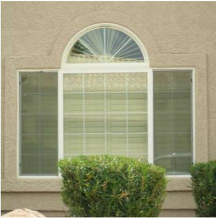
*Retrofit does not match existing frame dimensions and is not allowed*
