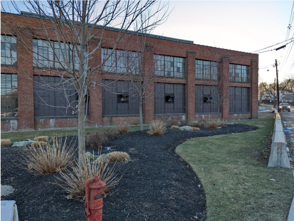
3.) Space Center, 83 Morse St. (3 of the brown panel frames)
