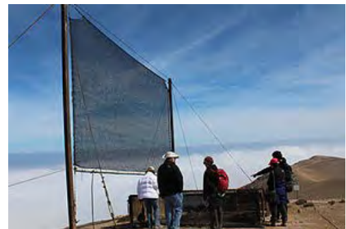
"Atrapanieblas" fog collection in Alto Patache, Atacama Desert, Chile
