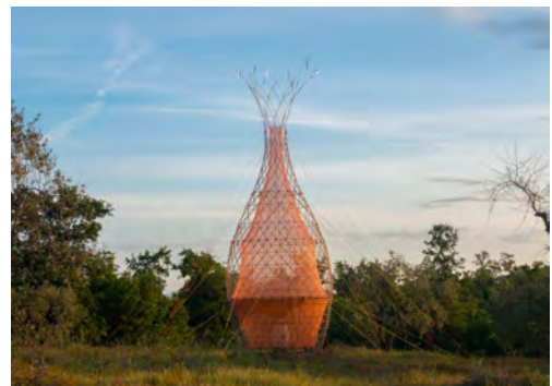
Warka Water Tower V1 Ethiopia
