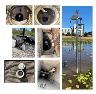
LIQUA-Level is a robust water-level measurement system for stormwater infrastructure.
