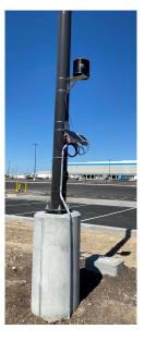
LIQUA-Level EPC is a robust water-level and sediment measurement system for stormwater infrastructure.
