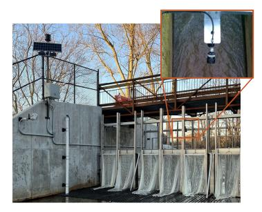
VELO is a robust flow velocity monitoring system for stormwater infrastructure.
