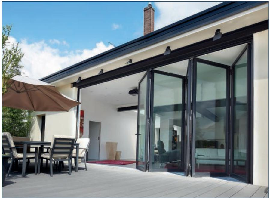
**FOUR (4) FT. WIDE DOOR PANELS.** Four (4) ft. wide panels improve sight lines and reduces the number of door sections, with a third less panels within a 12 ft. door opening compared to other solutions in the market.
