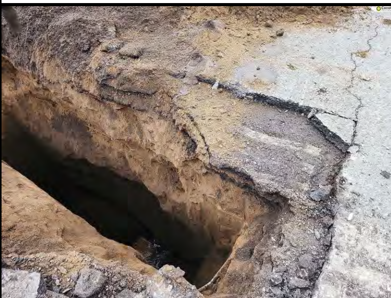
Exposed subsurface soil profile within test-pit TP-8
