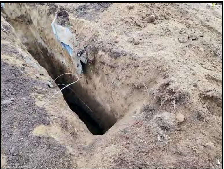
Exposed subsurface soil profile within test-pit TP-3
