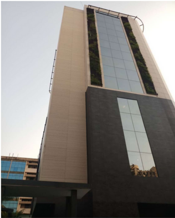
PROJECT: HAPPY HOMES, ANDHERI, MUMBAI , M/s. AJMERA BUILDERS ARCHITECT: M/s. REZA KABUL ,MUMBAI`` (STR. GLAZING, SPIDER GLAZING. LAMINAM CLADDING ,ALUMINIUM OVAL LOUVERS)
