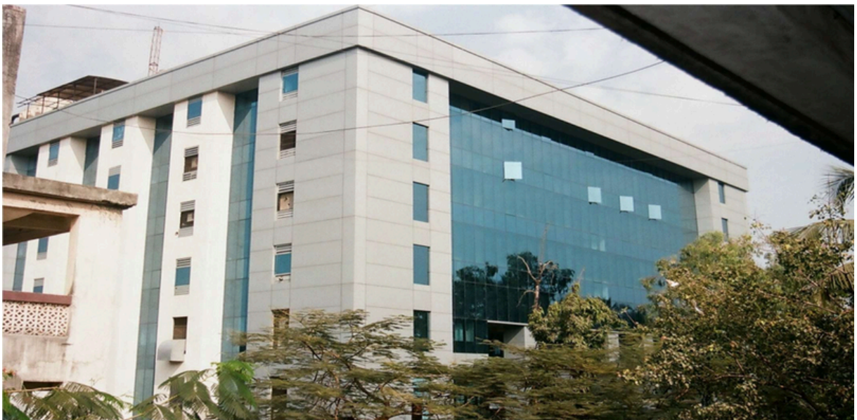
PROJECT: HAPPY HOMES, ANDHERI, MUMBAI , M/s. AJMERA BUILDERS ARCHITECT: M/s. REZA KABUL ,MUMBAI`` (STR. GLAZING, SPIDER GLAZING. LAMINAM CLADDING ,ALUMINIUM OVAL LOUVERS)
