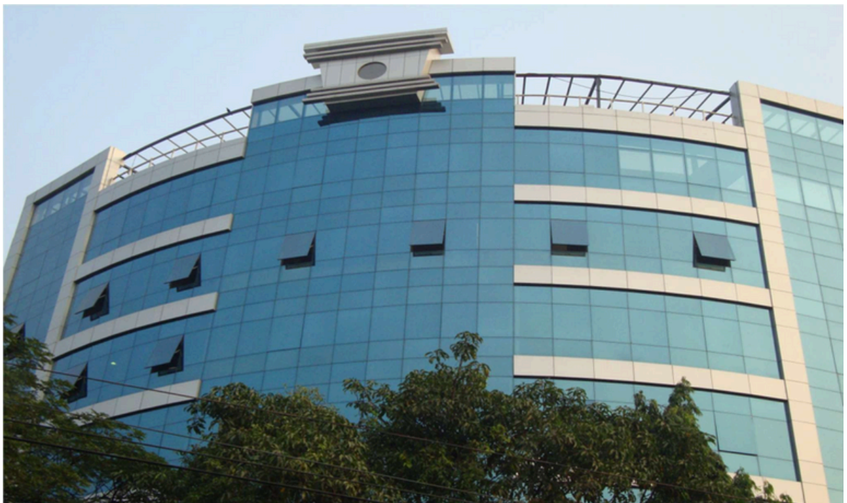
PROJECT: SANJAR ENCLAVE , MALAD, MUMBAI , M/s. SANJAR BUILDERS ARCHITECT: M/s. REZA KABUL ,MUMBAI (STR. GLAZING, SPIDER GLAZING. ACP CLADDING )
