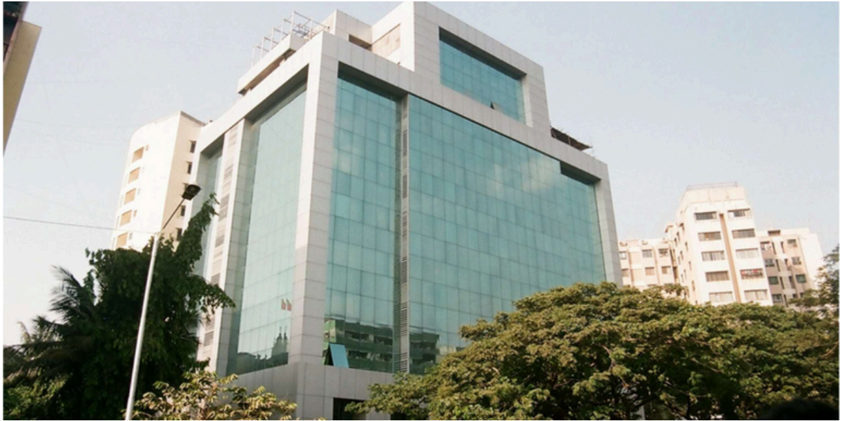
PROJECT: VIABHAV CHAMBERS, BKC , MUMBAI M/s. VICTORIA ENTERPRISES (PITTIE GROUP) ARCHITECT: M/s. KUTUB MANDIVALA (STR. GLAZING, ACP CLADDING )
