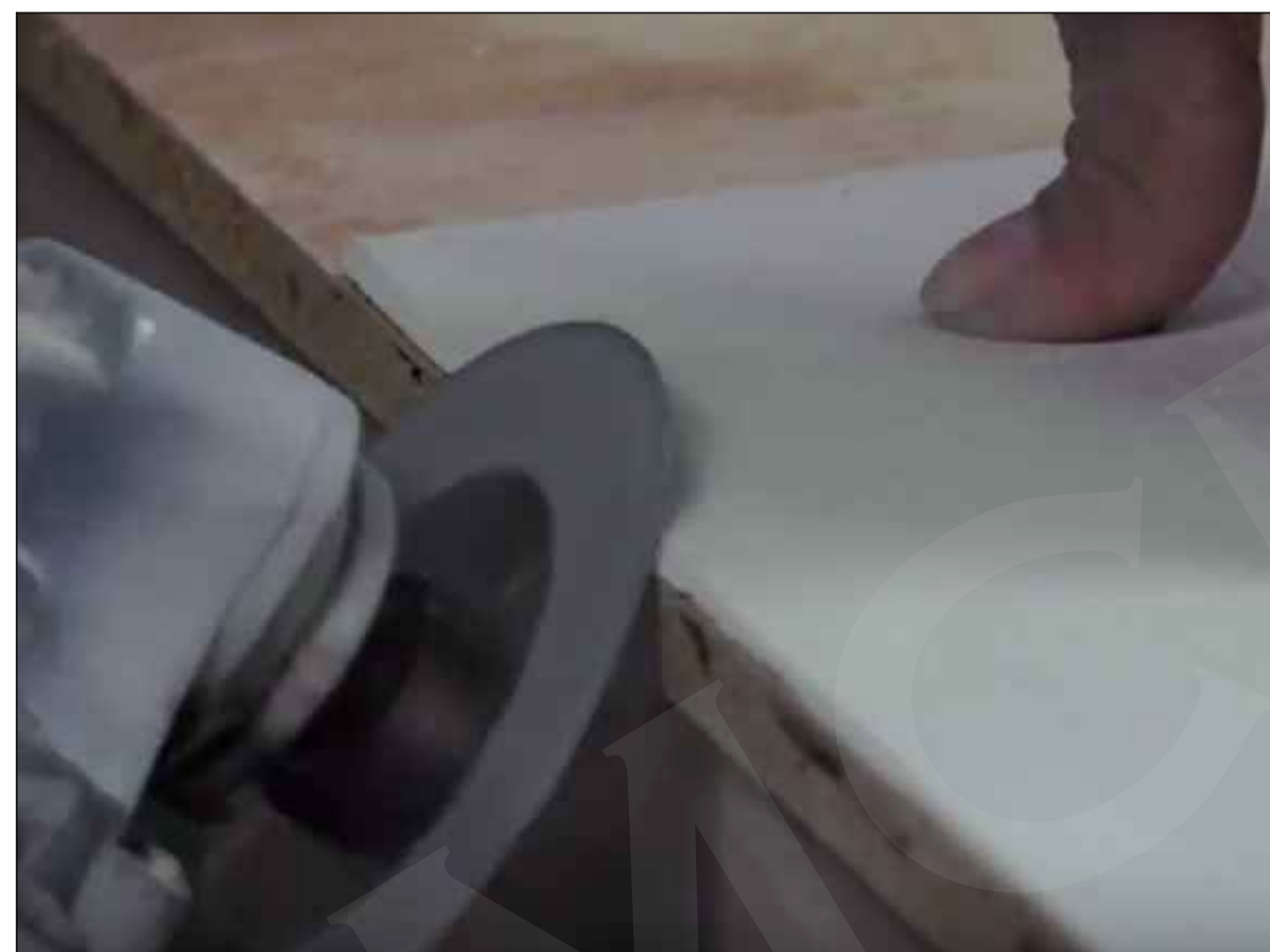
CHAMFERING OF SHEET EDGE WITH GRINDER
