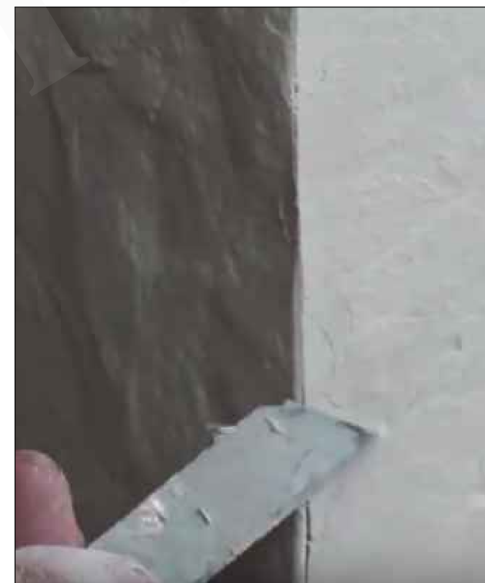
GROUTING AT THE JOINT
