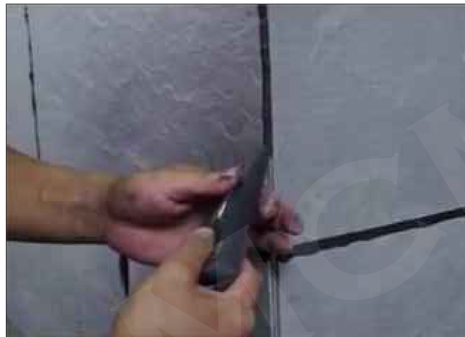
GROUTING AT EDGE
