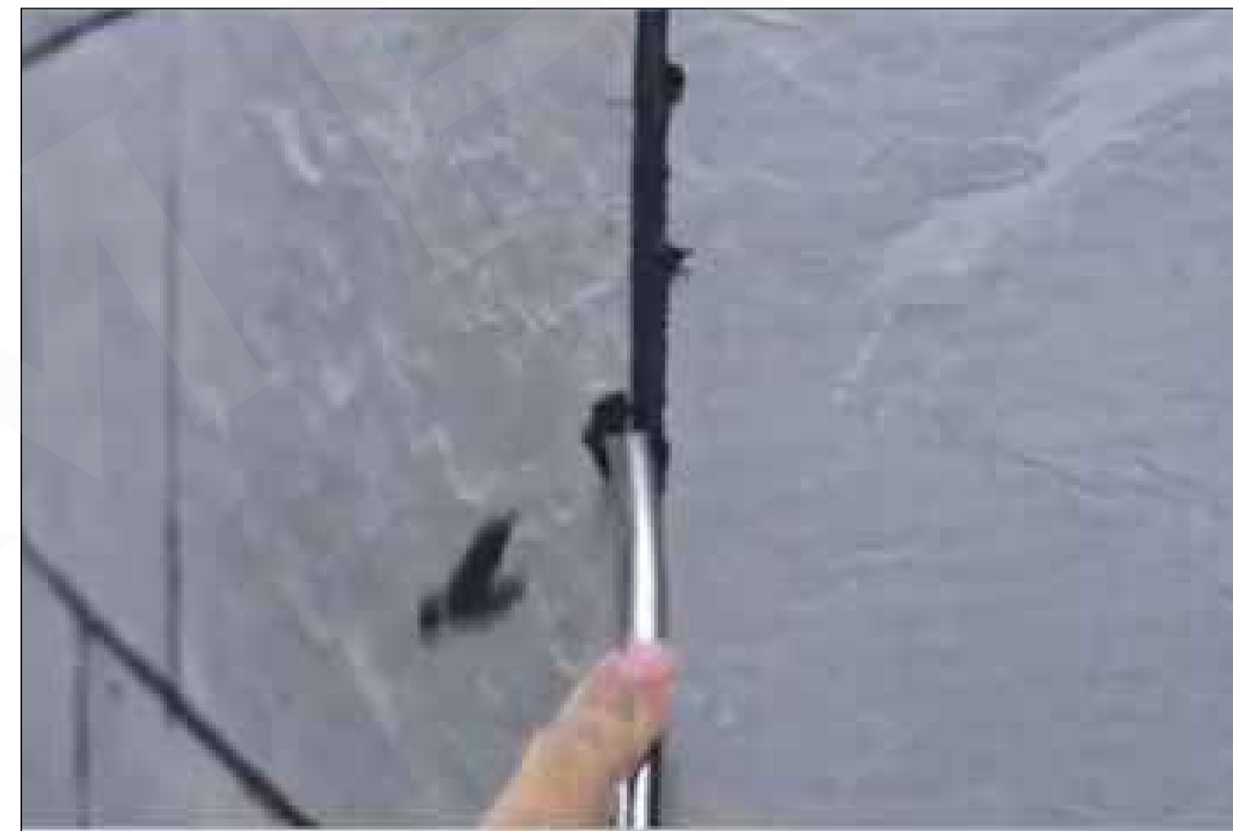
SMOOTHENING OF GROUTS AT EDGE
