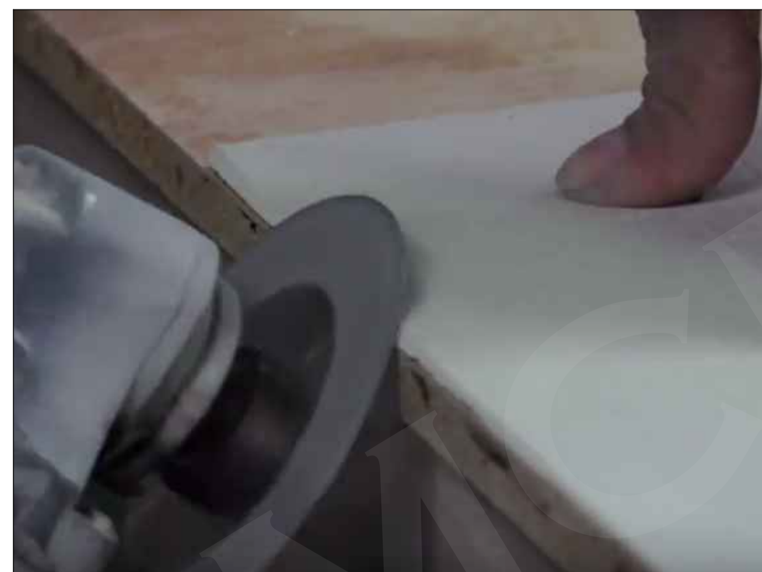
CHAMFERING OF SHEET EDGE WITH GRINDER
