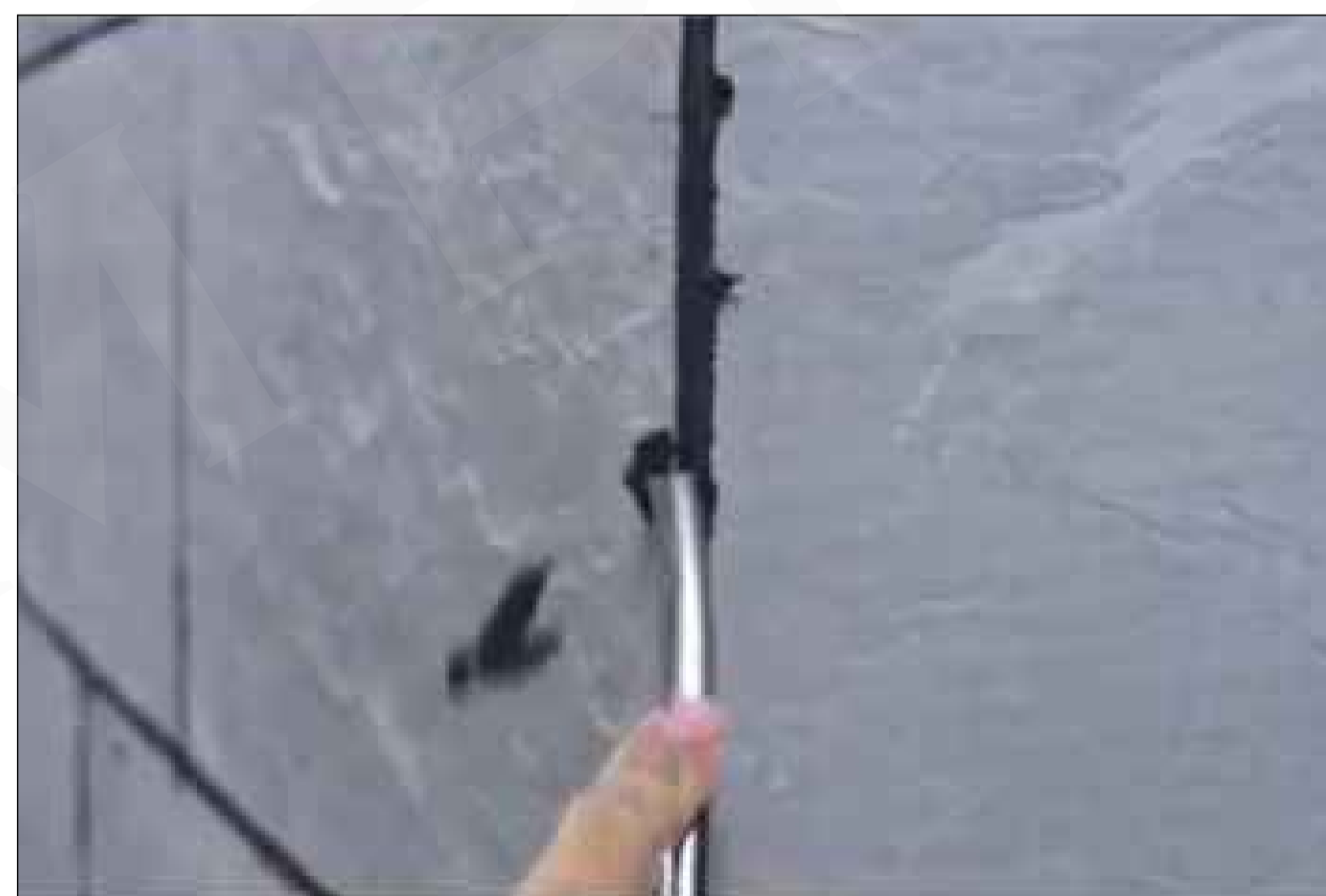
SMOOTHENING OF GROUTS AT EDGE
