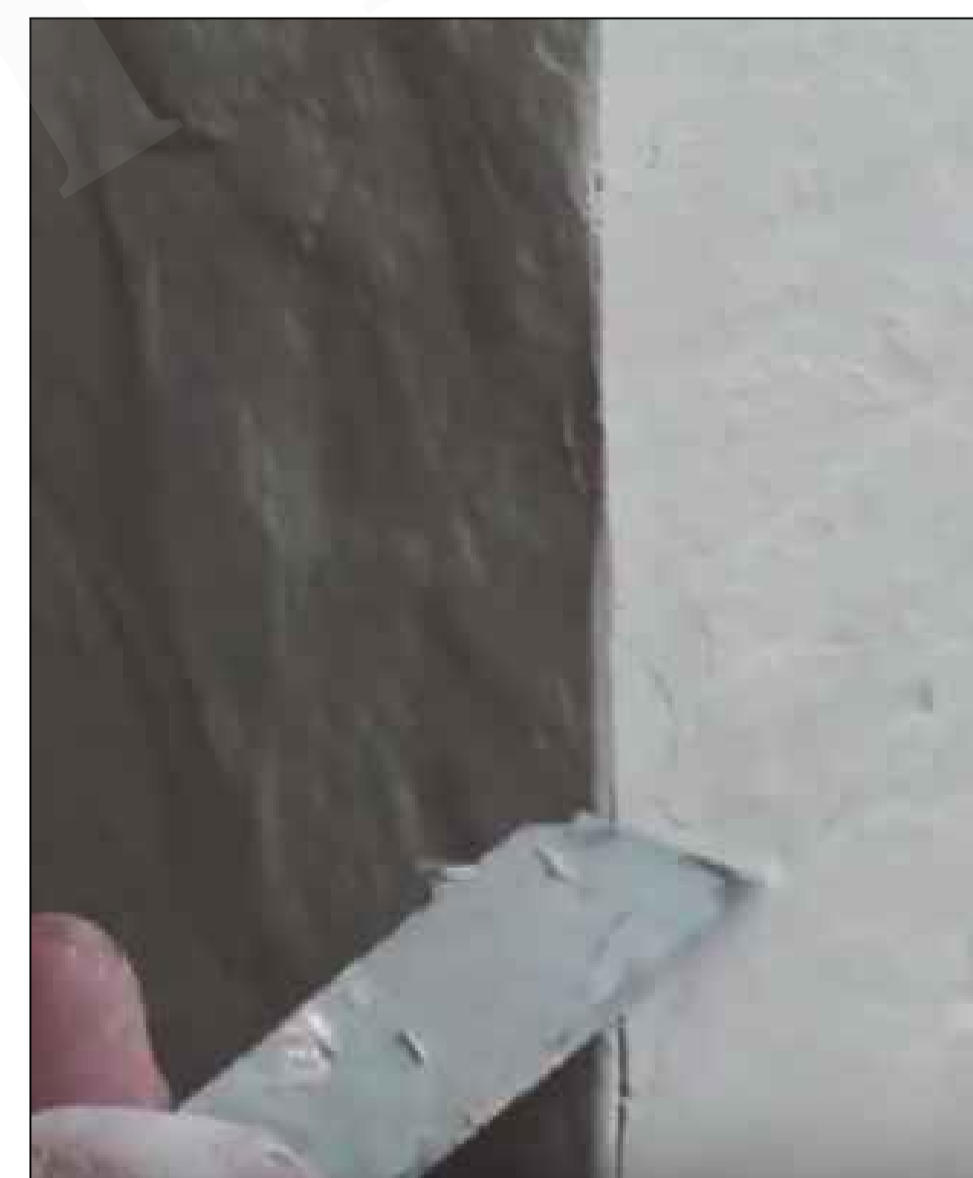
GROUTING AT THE JOINT
