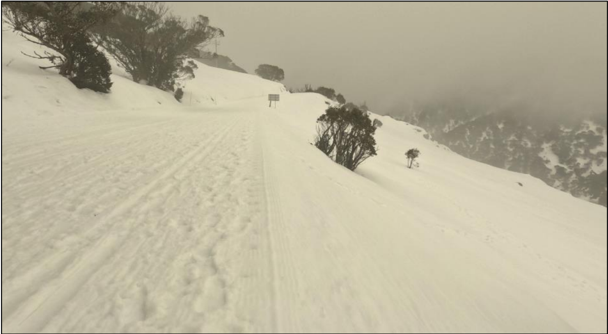
Approaching the bowl intersection looking back towards Falls Creek : showing the steep batter drop-off
