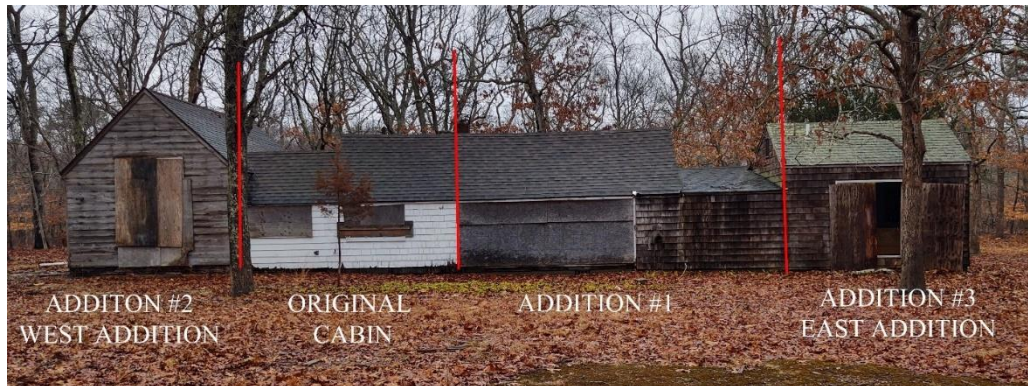
Photo No. 1: The residence as it stands today is comprised of four building campaigns starting with the original cottage moved to the site in the 1950s.
