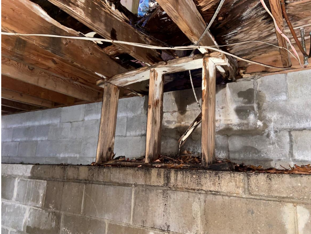
Studio floor frame rotted and temporary support rotted
