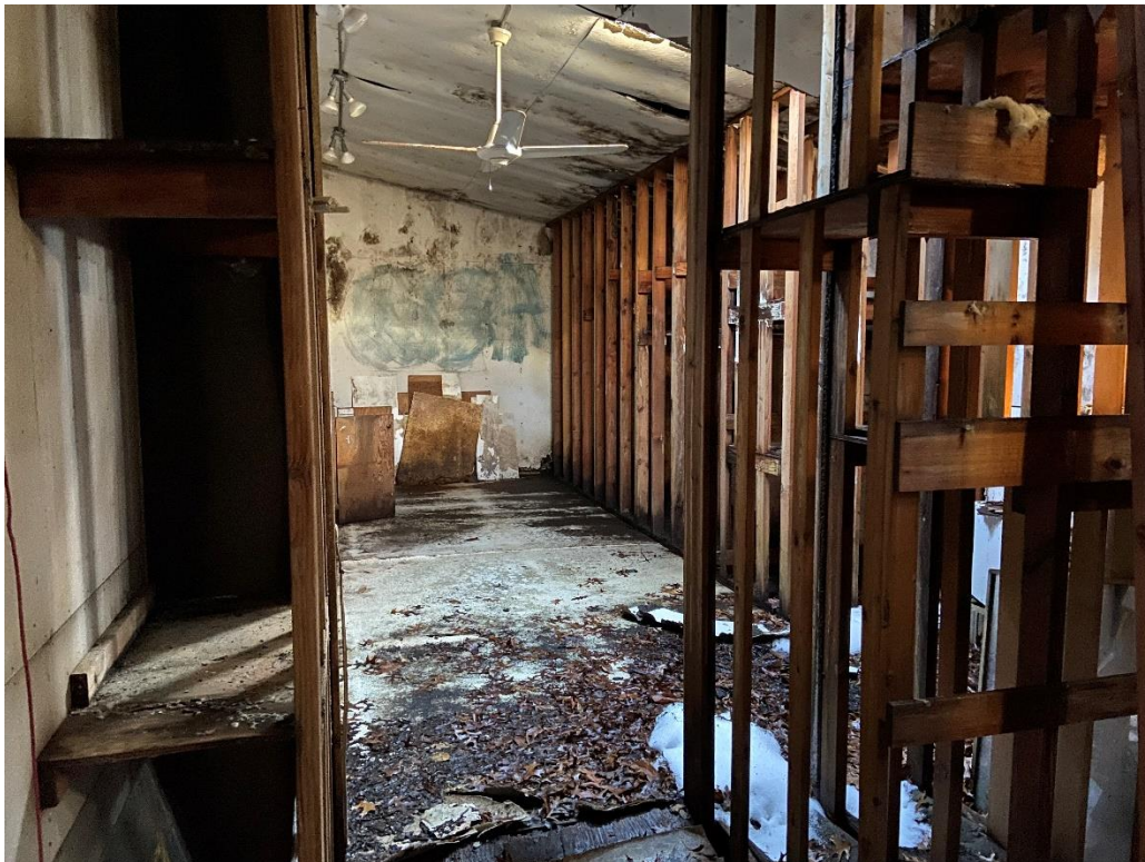
Studio storage area – daylight through roof
