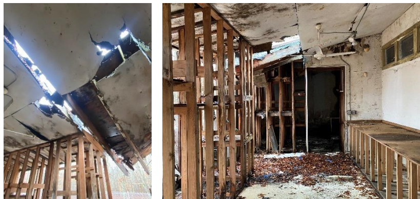
Photo No. 20 and 21: Ceiling and Wall finishes at the storage wing are heavily damaged from failure of the roof and rear wall.
