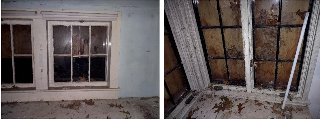
Photo No. 6 and 7: The windows all require some level of repair. While most only require re-glazing, some have damaged mullions requiring sash restoration.
