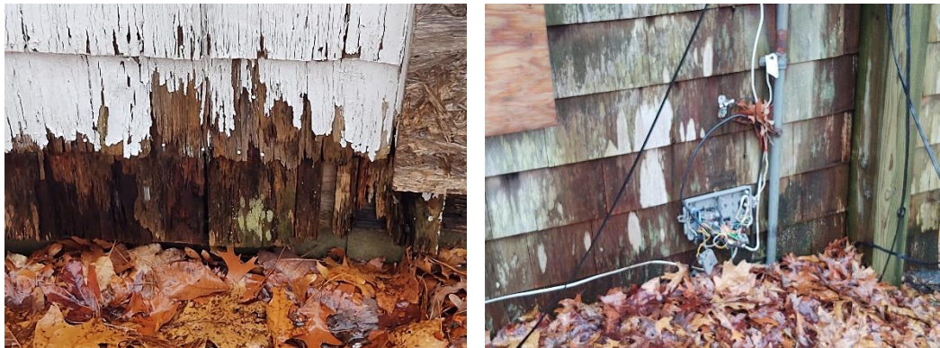
Photo No. 4 and 5: Minimal roof overhang, excessive soil overburden, and accumulated organic detritus are all contributing to cladding damage at the residence.
