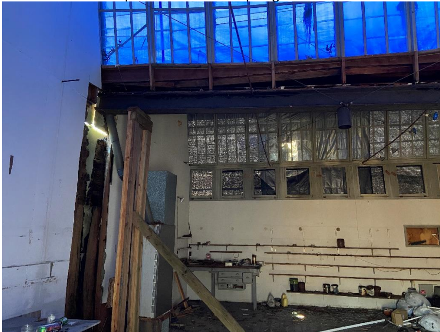
Brooks Studio Parapet roof beam collapsing
