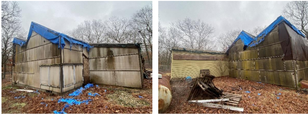
Photo No. 14 and 15: The Brooks Studio was built over two campaigns, the main block clad in Transite panels, and the SE storage wing clad in aluminum siding.
