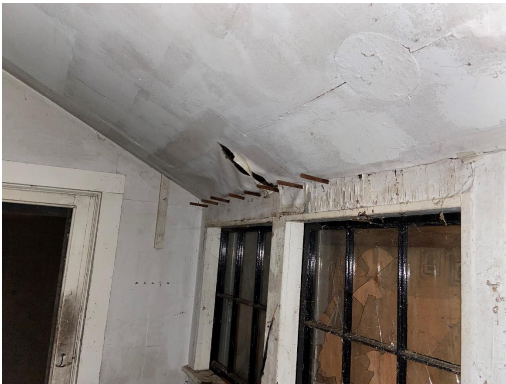
Roof leak above kitchen
