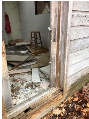
Photo No. 24 and 25: The window sash and frames are salvageable but will require re-glazing. The entry door is heavily damaged and will require full restoration.
