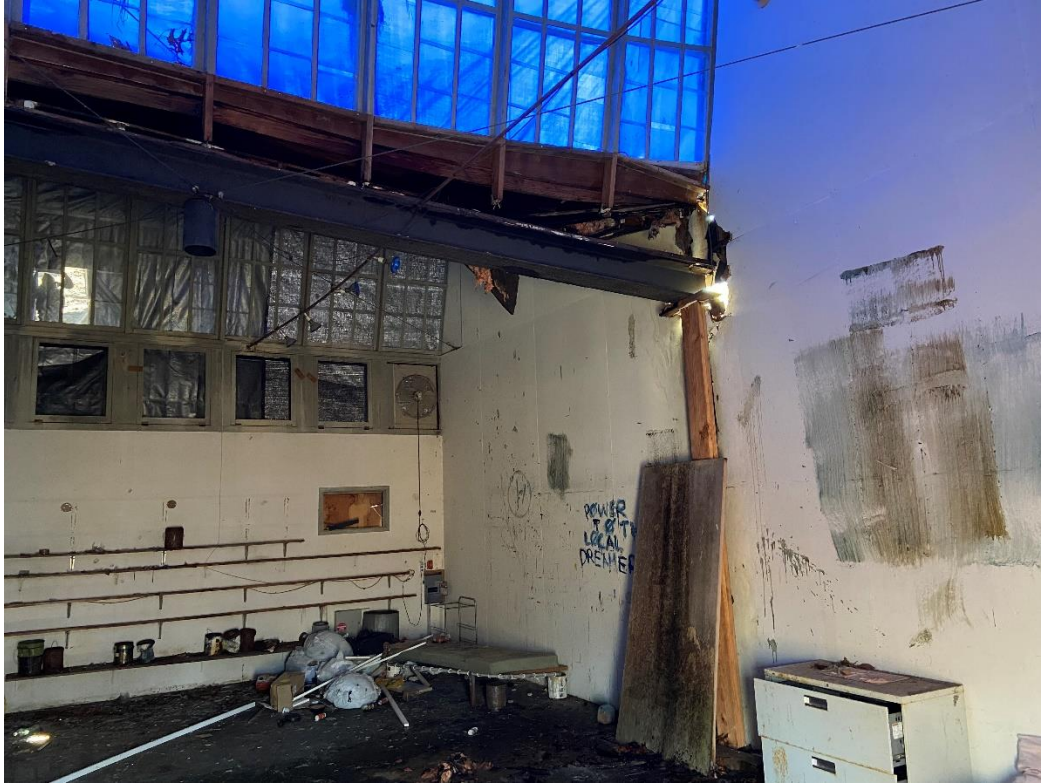
Brooks Studio Parapet roof beam collapsing
