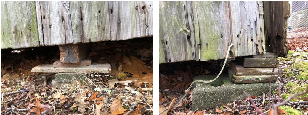
Photo No. 30 and 31: The foundation elements do not properly support the structure.
