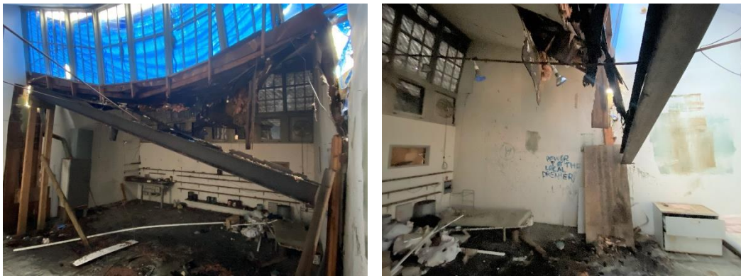
Photo No. 18 and 19: Chronic water infiltration has resulted in significant damage to the roof and skylight.
