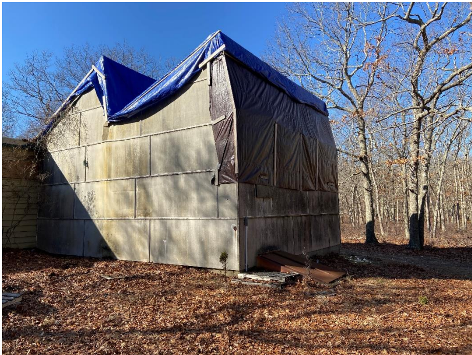
Studio roof leaking through tarp, upper walls are twisting and buckling
