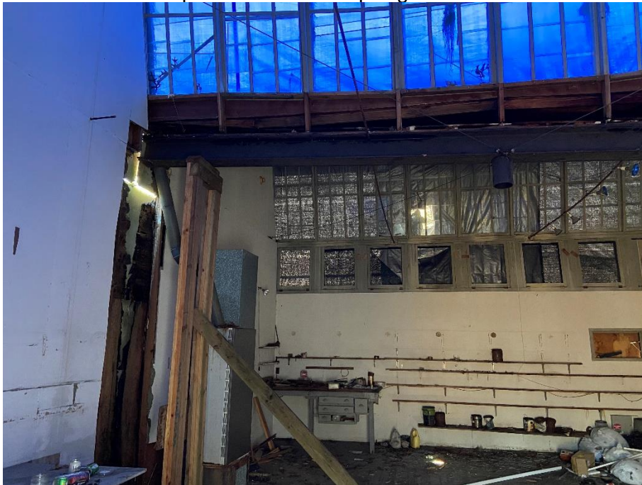
Brooks Studio Parapet roof beam collapsing
