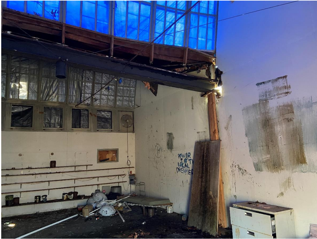
Brooks Studio Parapet roof beam collapsing
