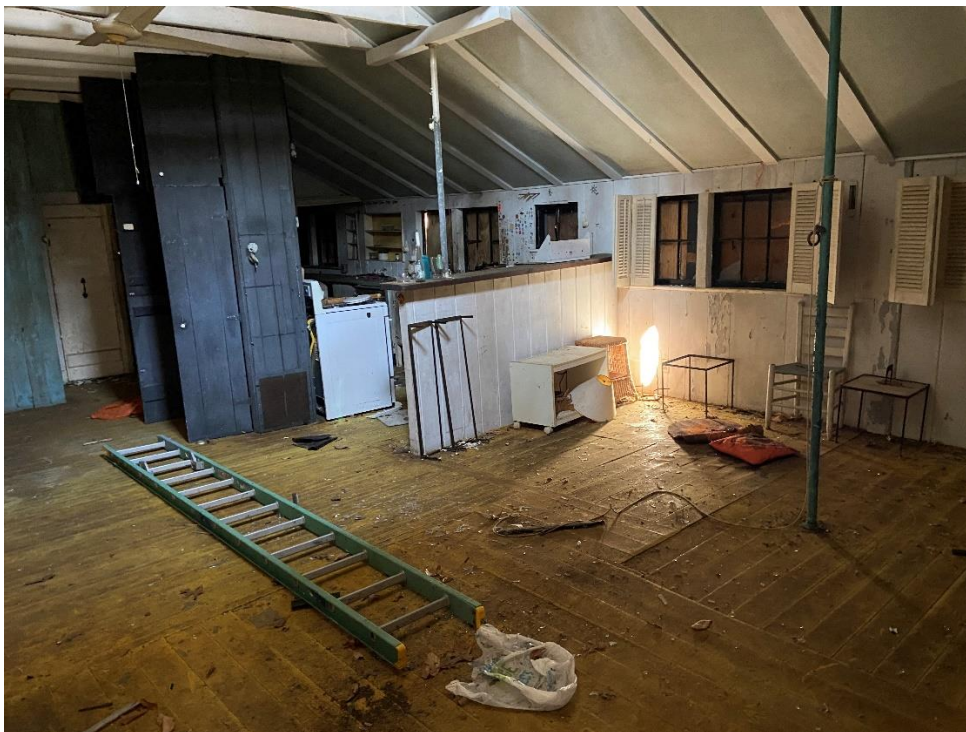
Cottage interior..center column is punching through the floor due to rot. Beam at roof is rolling
