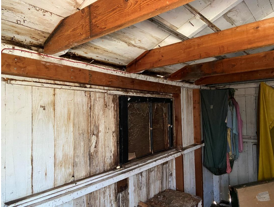
Inside shed, water penetration, sheathing rot
