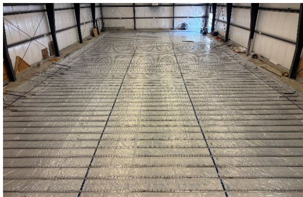
“Chairs” positioned on poly layer
