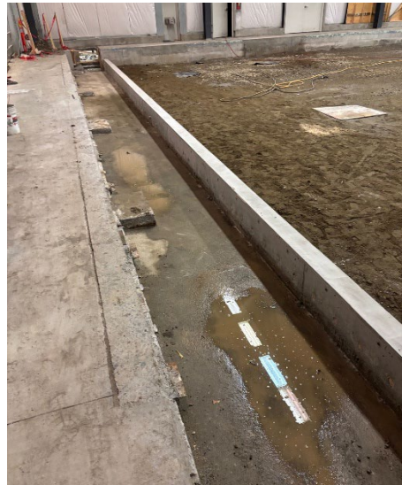
New header trench wall
