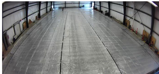
Insulation complete. 2 nd poly layer installed.
