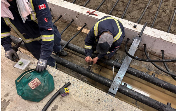
Connecting (“fusing”) glycol lines to header
