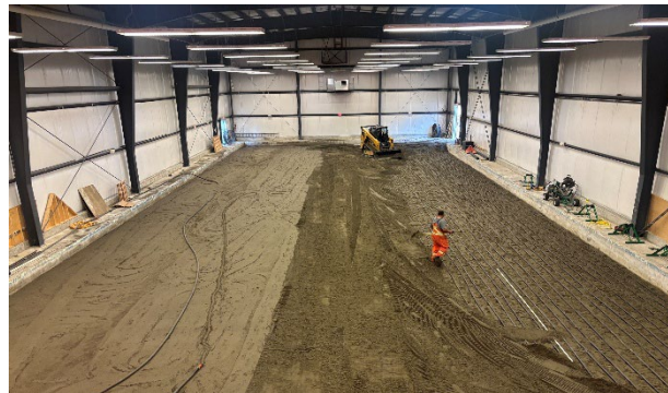
Tamped sand layer on left. Sand addition underway on right.
