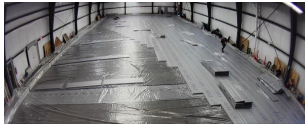
Installing 1 st insulation layer on first poly barrier
