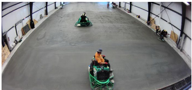
Finishing (power troweling) (1pm)
