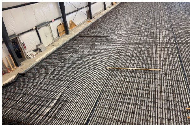
Brine lines placed into position
