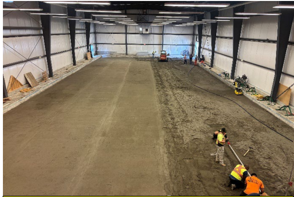
Manually leveling the sand layer
