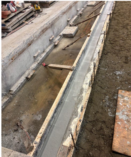
New header trench wall poured
