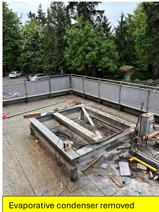
Removing the chiller
