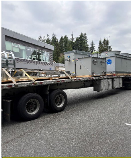
Evaporative Condenser delivery
