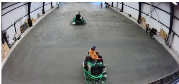
Finishing (power troweling) (1pm)
