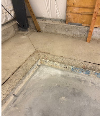
Slab perimeter caulked/sealed
