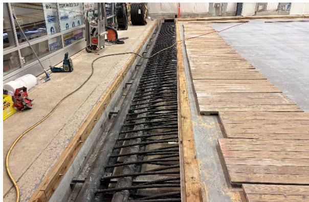
(Old) trench covers being re-fitted
