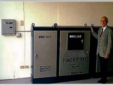
Cabinet on left will house 26.4 kWh Lead Cobalt Battery (240-volts @ 110-amps I/ C) Cabinet in center will house 15.8 kW Fuel Cell (288-volts @ 0.8 volts' cell under 55-amp load) Cabinet on right will house DCto ACInverter,
