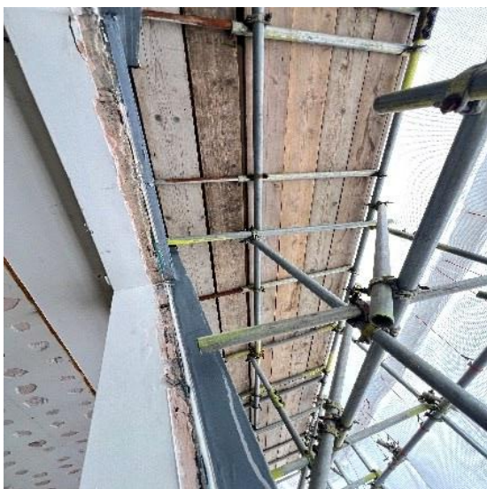
Two-level debris protection and local guarding
