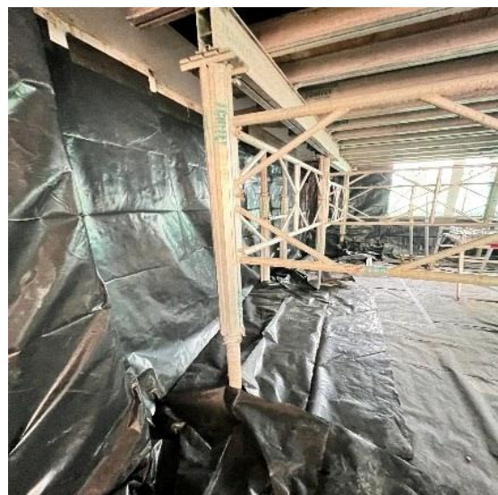
Temporary weathering to exposed party wall areas
