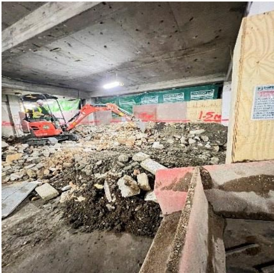
Basement piling activity within constrained working area
