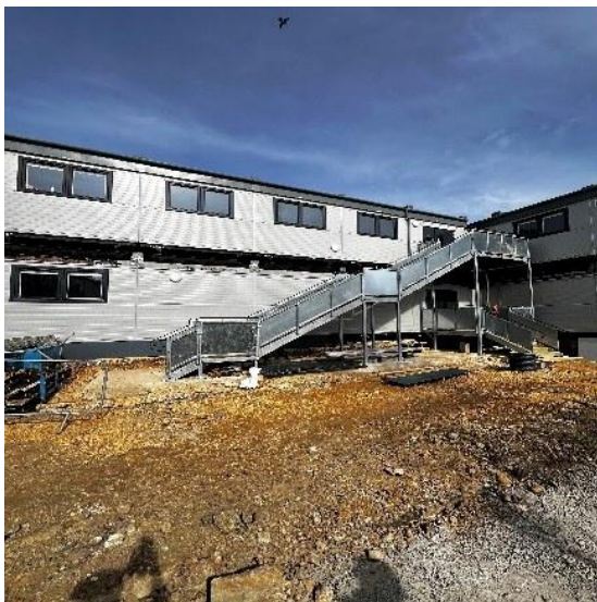
Temporary modular accommodation and external works interface
