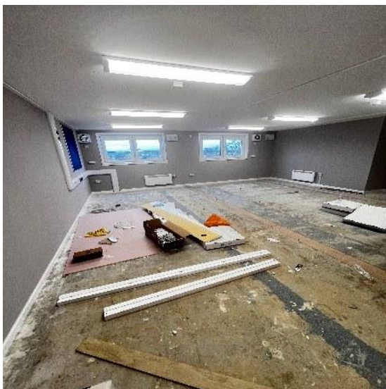
Internal fit-out progress within temporary accommodation
