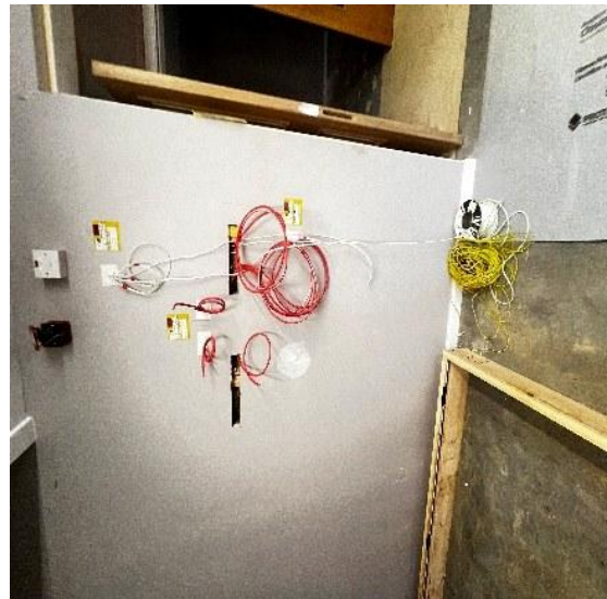
Second fix services and fire stopping coordination zone
