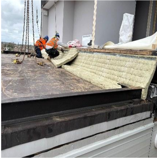
Fire barrier installation at modular roof interface
