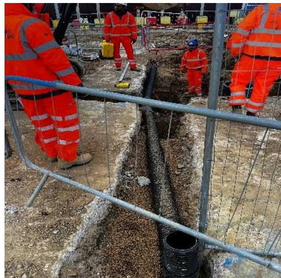
Below-ground services and segregated excavation zone
