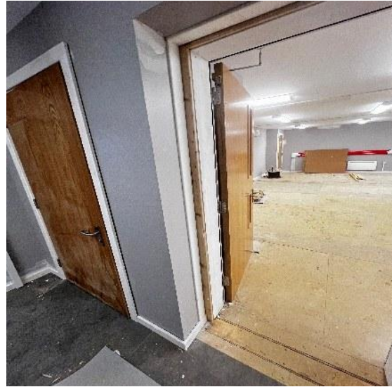
Fire door and modular junction interface under review
