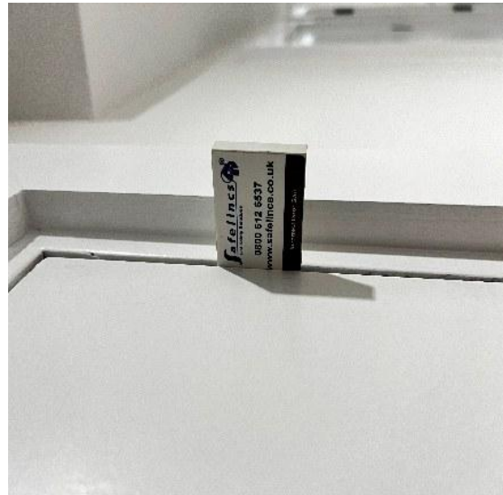
Fire door label and closer review
