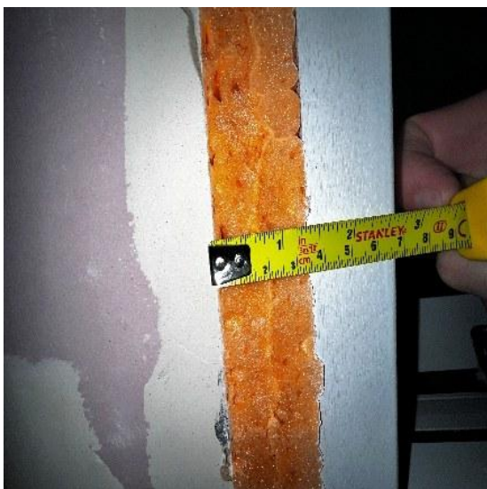
Linear gap check within riser location
