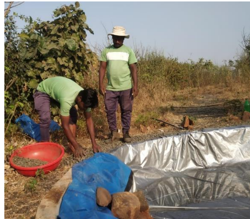
Figure 24: Adding pond liner
