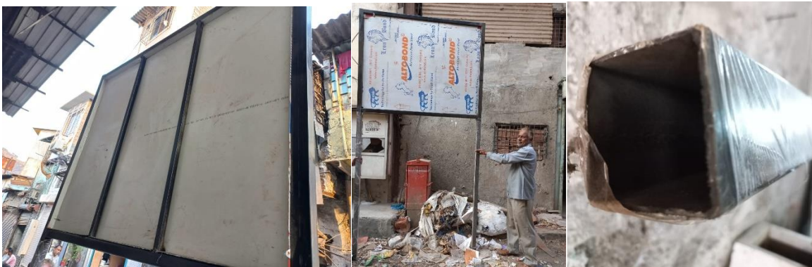
Figure 35: Fabrication work of Exhibits
