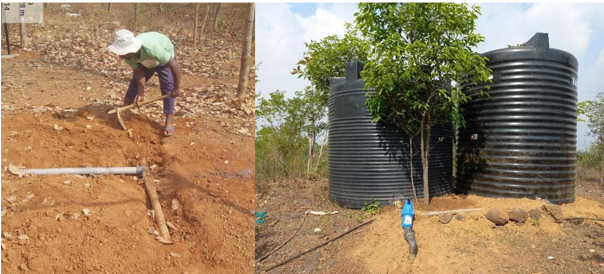
Figure 16: Dripline work connecting water tanks
