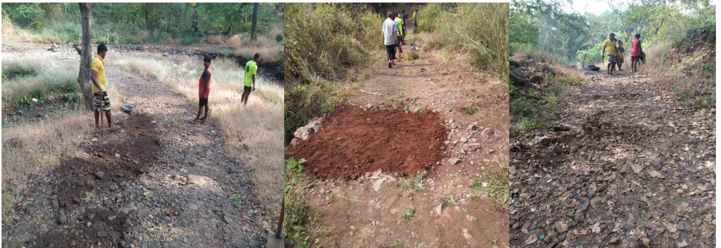
Figure 10: Repairing of road
