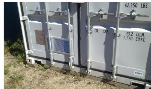
Figure 12 Explosion-Relief Panels, Delcourt & Garis, (2014) P.10 [27, p. 16]
