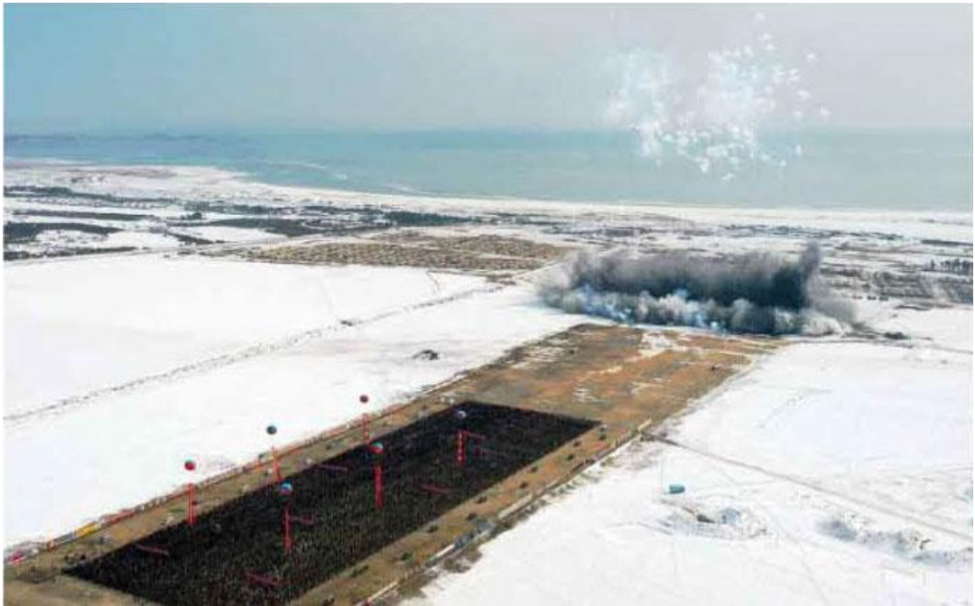
First blasting in the Ryonpho area 230-odd days ago
