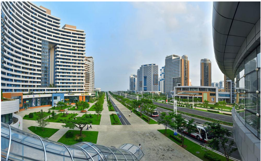
The viaduct linked to sidewalks
