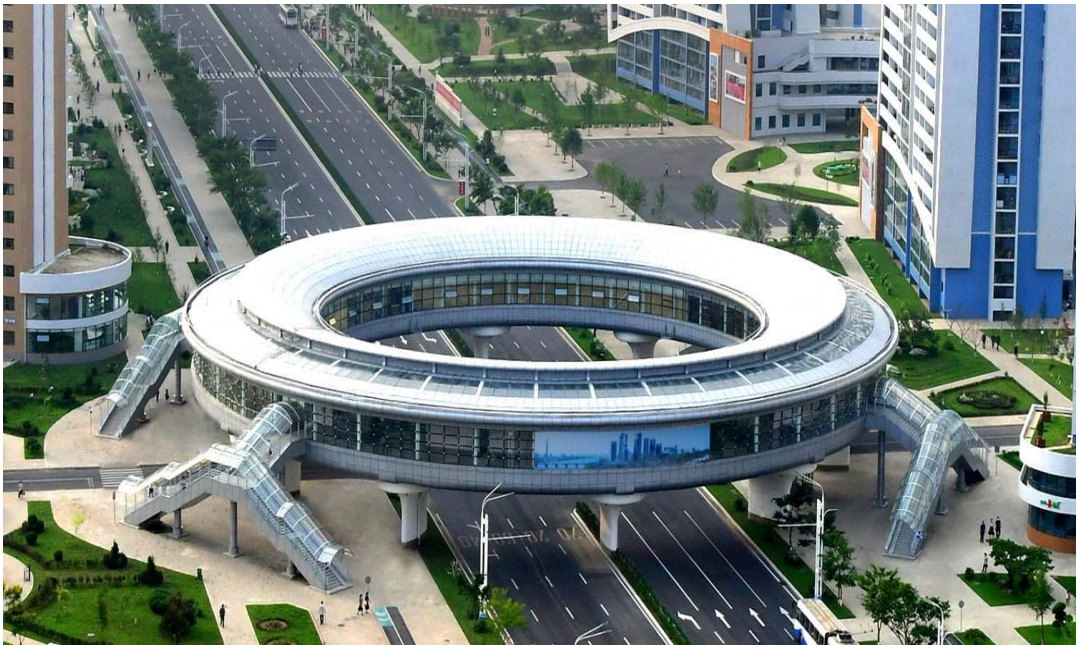
The viaduct in Songhwa Street
