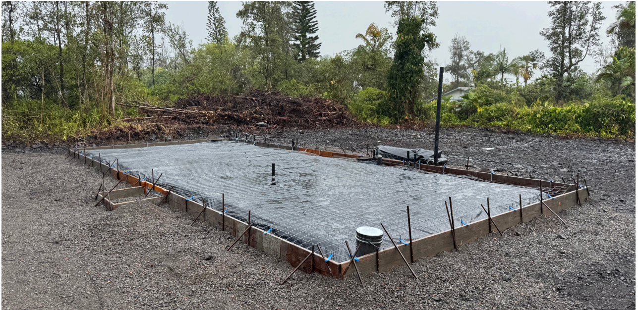
Foundation formed up. Plumbing, and electrical work has passed inspection. Ready to pour concrete
