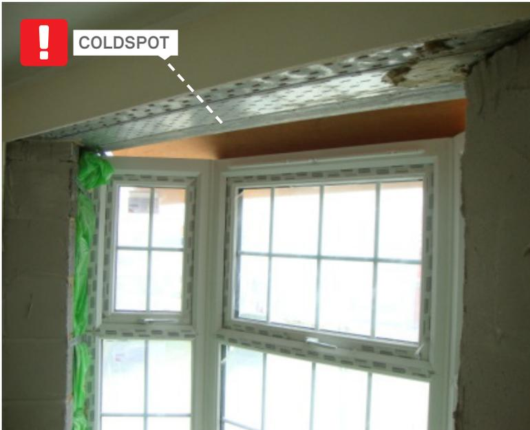
THICK FRAME AND POSTS INCREASES HEAT LOSS
