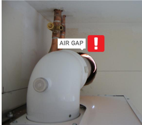
BOILER FLUE NOT SEALED
