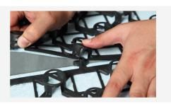
4) Lay the pipes (it may be necessary to use some R983Y041 plugs for pipe anchorage).
