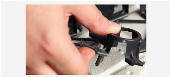
c. for codes R979SY021 and R979SY025, position the panels on the foundations or existing floor, overlapping the side couplings to ensure each panel is interlocked with the next one (it may be necessary to use some R983Y040 plugs to make sure the net adheres to an existing floor).
