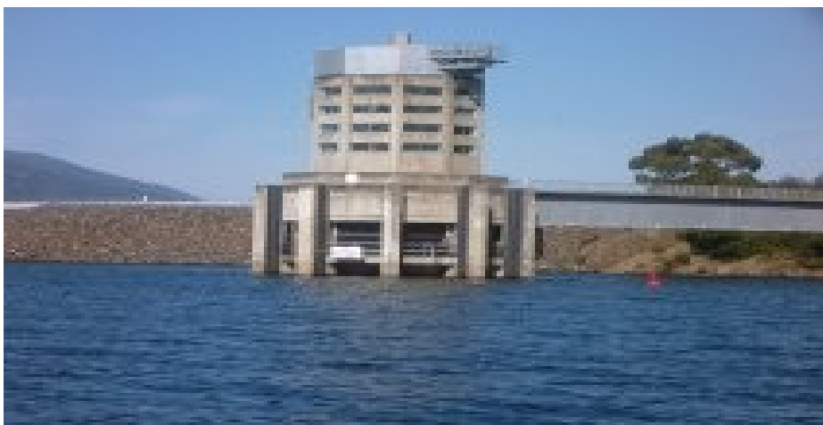
Eildon Wall and Control Tower
