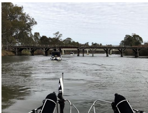
Figure 7 - Goulburn River heading upstream under Chinaman's Bridge
