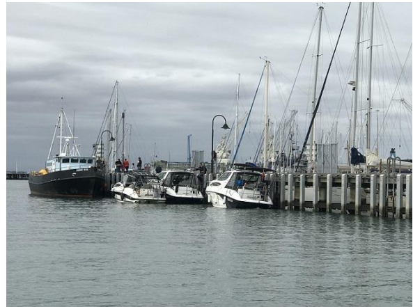
Figure 15 - Williamstown Public wooden Jetty
