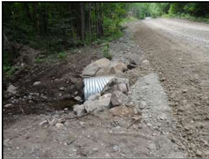
Figure 3. Excellent water crossing on road construction on the Murphy Road.
