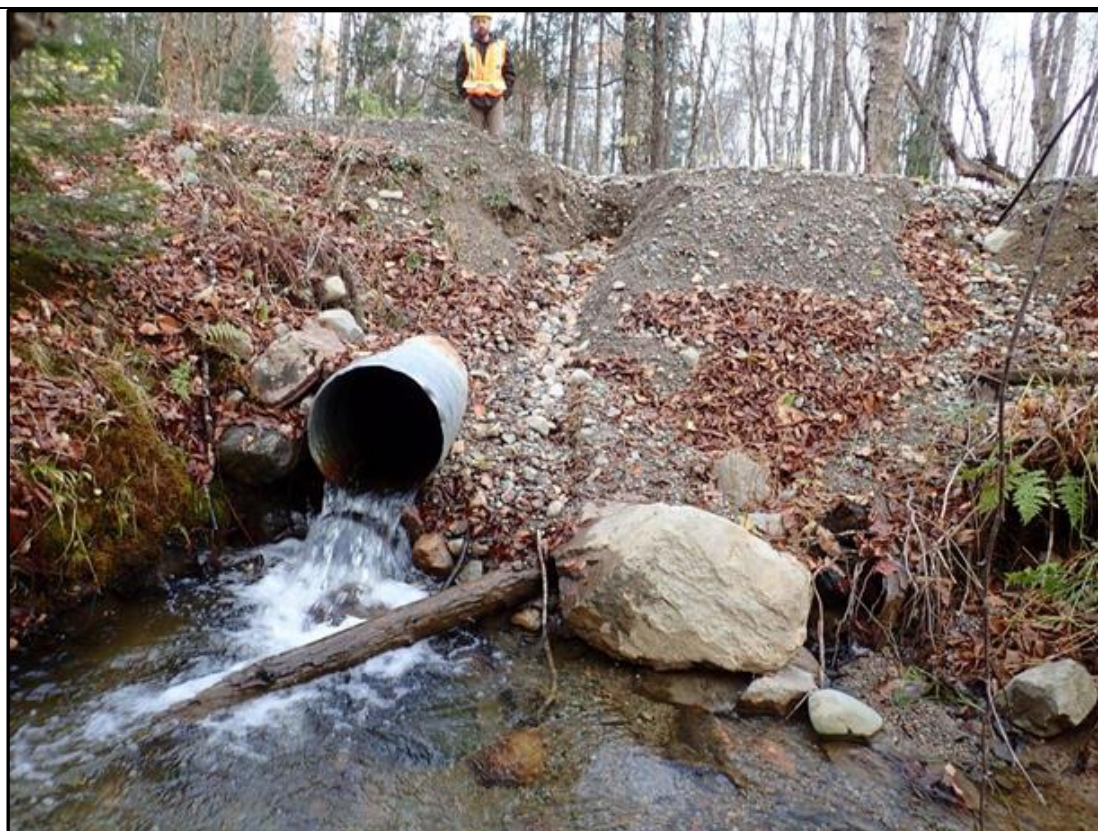
Figure 5. A perched and unstable culvert on the Jarvis Block.
