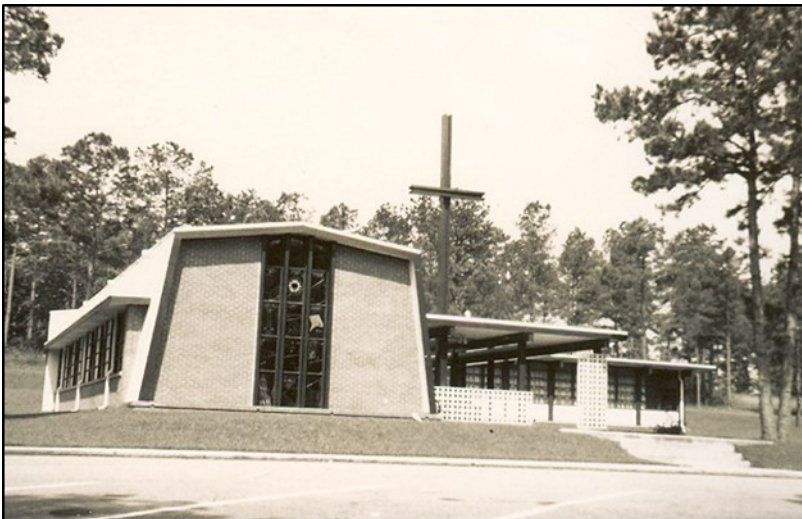
The photo looks pretty ancient, doesn't it? This building was built in 1961 – five years after St. Stephen was officially established.
