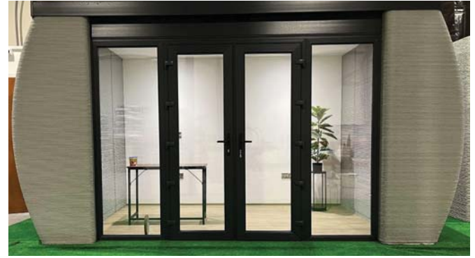
BELOW: The 'Versarien Lunar' pod – the world's first 3D-printed concrete product enhanced by graphene.
