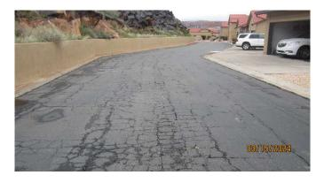
This is for the cleaning and sealing of cracks. We have budgeted for repairs which includes surface patch, crack repair and asphalt joint seal. This component is important in that it will extend the life of the asphalt if it is completed in a timely manner.
