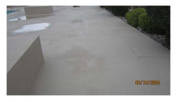
Per info sheet the pool deck was resurfaced in 2022. We have budgeted for resurfacing in 2040. Multi coat Kool Krete and 2 coats of BUFF urethane colorseal. 4,352 sq. ft.
