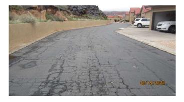
This is for the cleaning and sealing of cracks. We have budgeted for repairs which includes surface patch, crack repair and asphalt joint seal. This component is important in that it will extend the life of the asphalt if it is completed in a timely manner.
