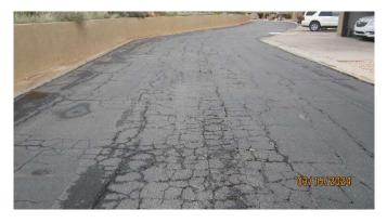
It will be necessary to adjust manhole and valve covers at the time the overlay is applied. Deflection testing should be conducted by an independent consultant near the end of the estimated useful life to determine the condition of the asphalt and estimated remaining life before the overlay is required.
