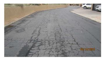
It wiill be necessary to adjust manhole and valve covers at the time the overlay is applied. Deflection testing should be conducted by an independent consultant near the end of the estimated useful life to determine the condition of the asphalt and estimated remaining life before the overlay is required.
