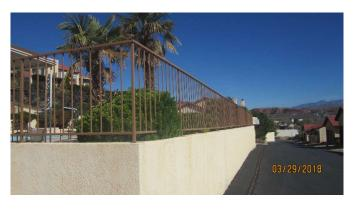
Stucco paint and repairs around the pool area have a useful life of 12 to 18 years. We have budgeted the paint and repairs for 2030. 4 pillars and 1,500 sq. ft. of stucco wall.
