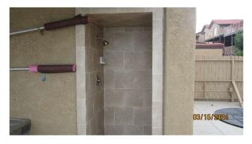
Tile walls and flooring will need to be replaced in the outdoor shower located outside the clubhouse. Per HOA notes all the fixtures and tiles with the shower were replaced in 2022 at a cost of \$4,000. 224 sq. ft
