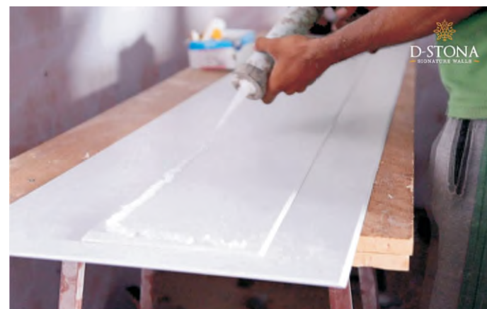
Sheet pasting using adhesive.
