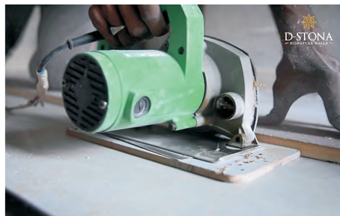
Sheet cutting using a hand cutter.
