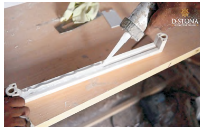
Molding pasting using adhesive.
