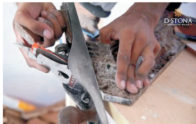
Molding joint surface planing using a planar knife.
