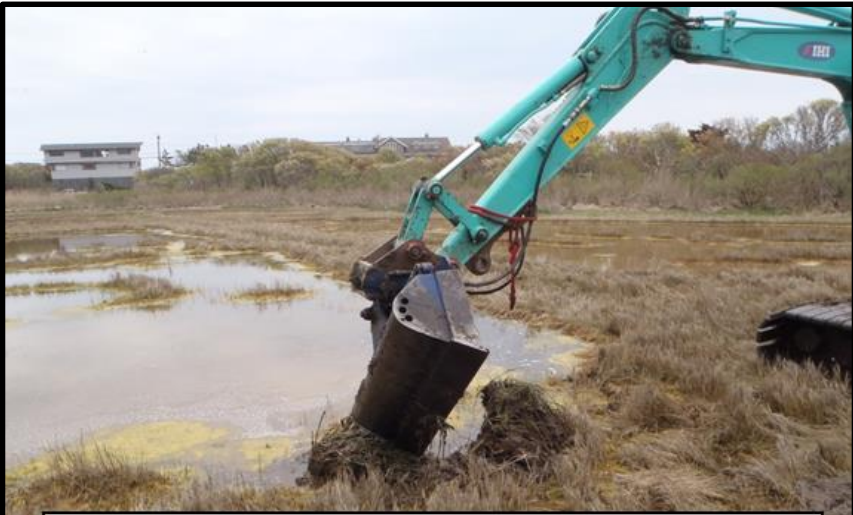
Runnels dug through ditch spoils
