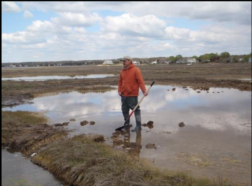
Runnels dug through ditch spoils
