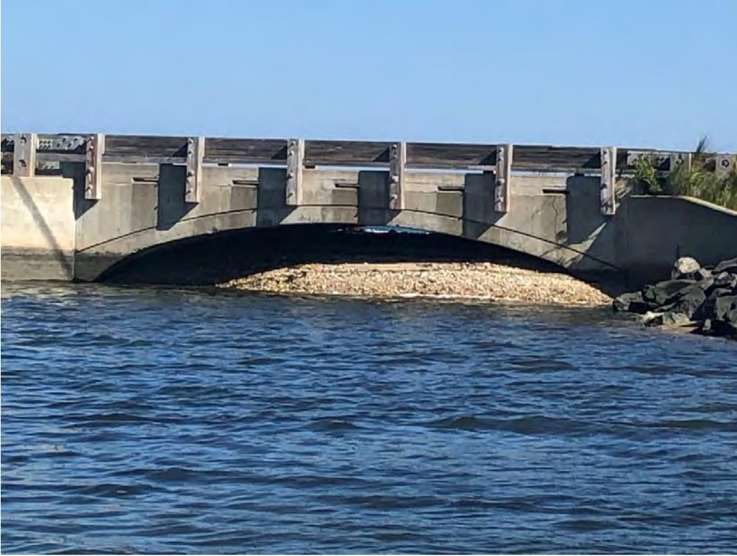
**Figure 10:** Photo taken on Oct 14<sup>th</sup> 2021 of closed culvert.
