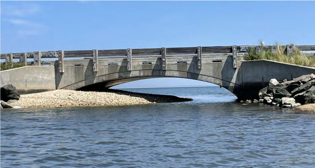
**Figure 12:** Photo taken on August 9<sup>th</sup> 2022 of partially closed culvert.
