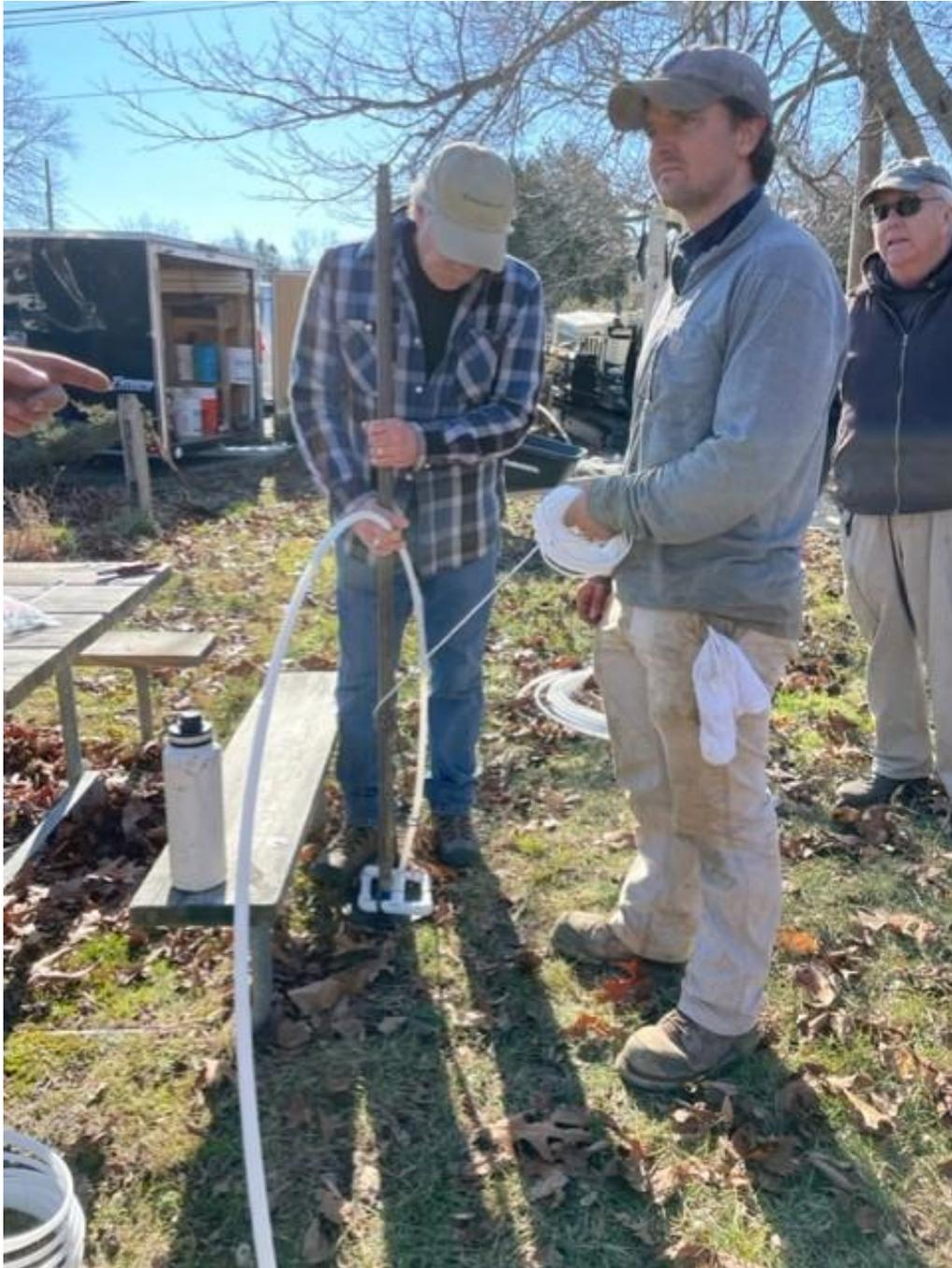
**Figure 3:** Photo of the air injection line before it was lowered into the bottom of the gravel column.
