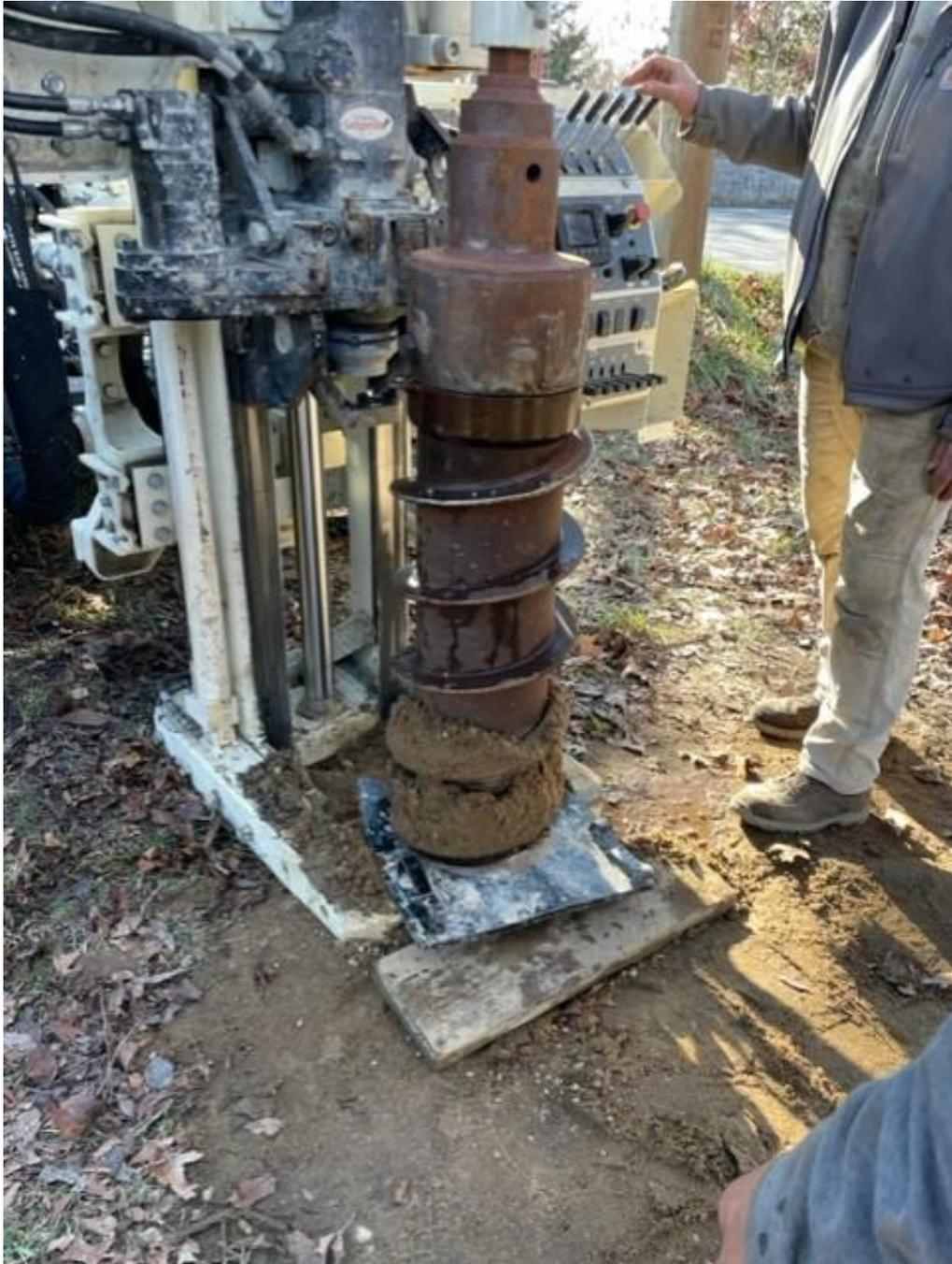
**Figure 2:** Photo of hollow stem auger drilled into the ground to create a ~1ft diameter by 30ft deep column which was then filled with gravel as well as an air injection line and sampling ports.
